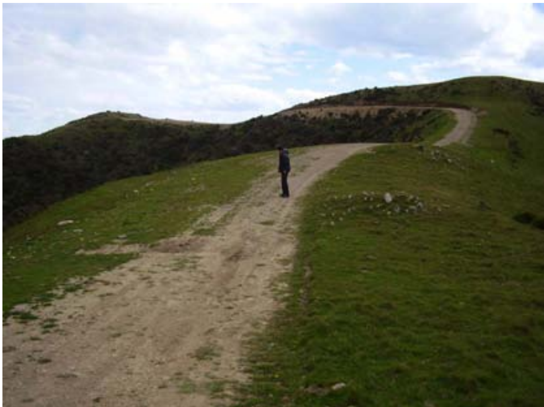
Site 23 – looking south-west with turbine location about 5m from author on left of track
