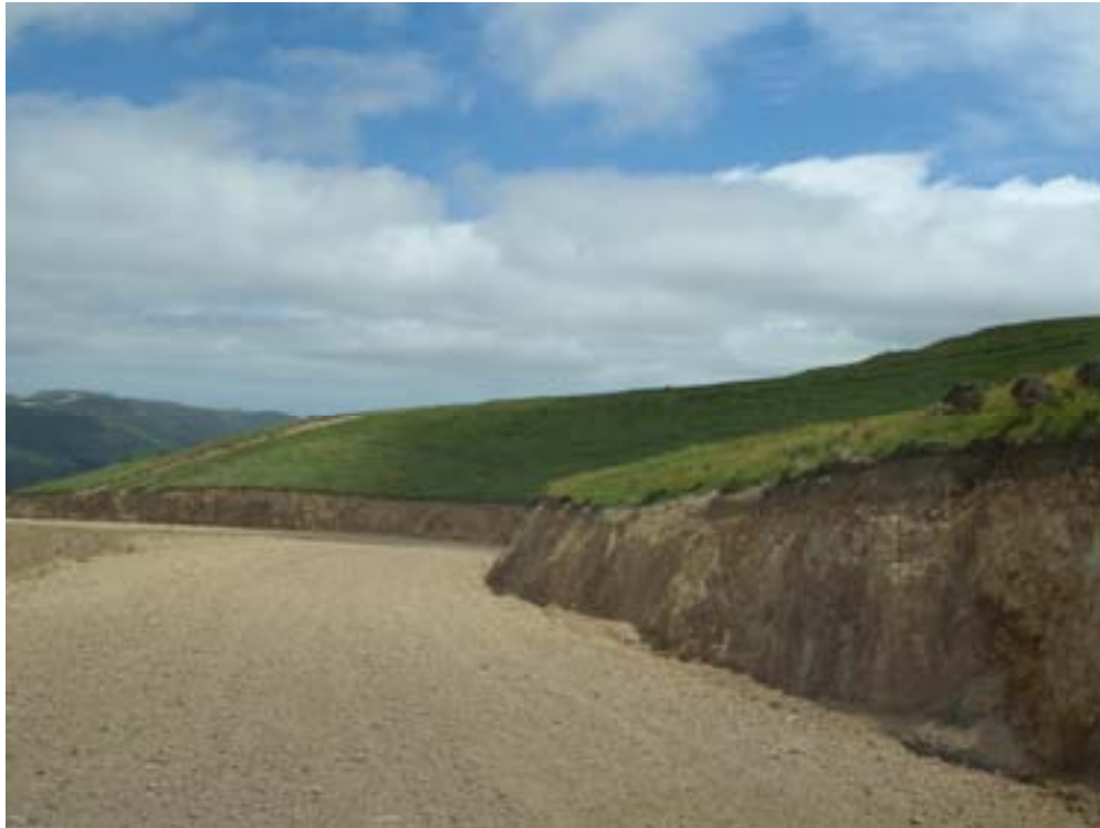
PHOTO 11 – Site of Turbine 26
