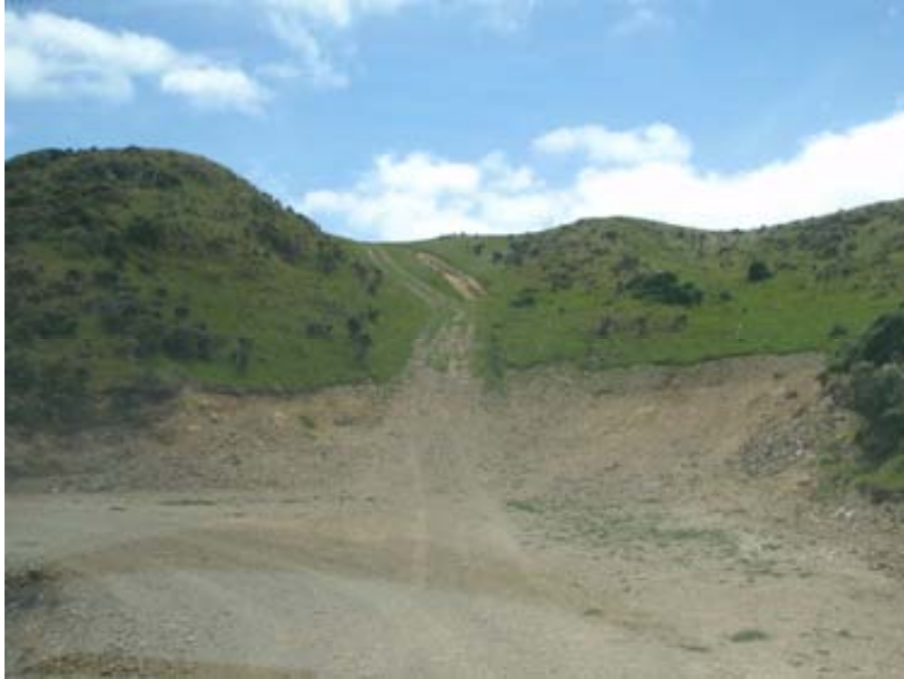
PHOTO 13 – Track access to Turbine 20 – Too steep, alternative route sort
