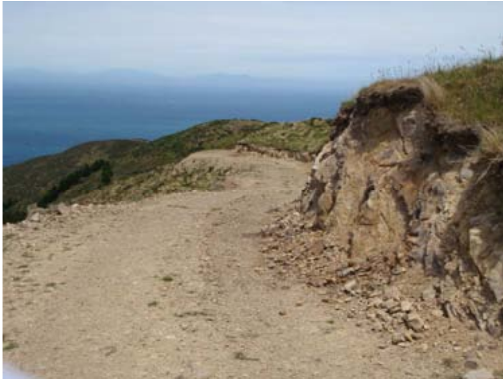
PHOTO 25 – Minor cut back required on RHS of main track for truck access
