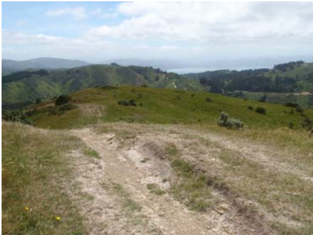
PHOTO 16 – Site of Turbine 19 - Earthworks of vertical alignment required
