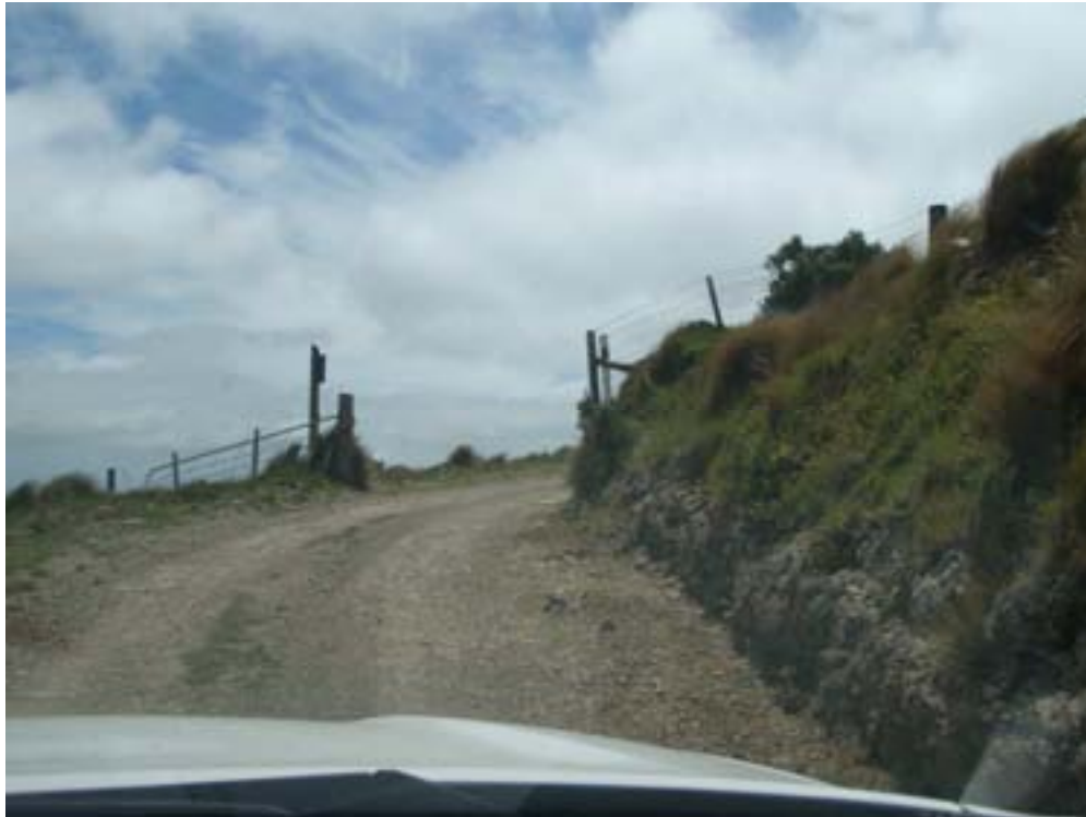
PHOTO 38 – 4 to 5m cut back required on RHS of main track for truck access
