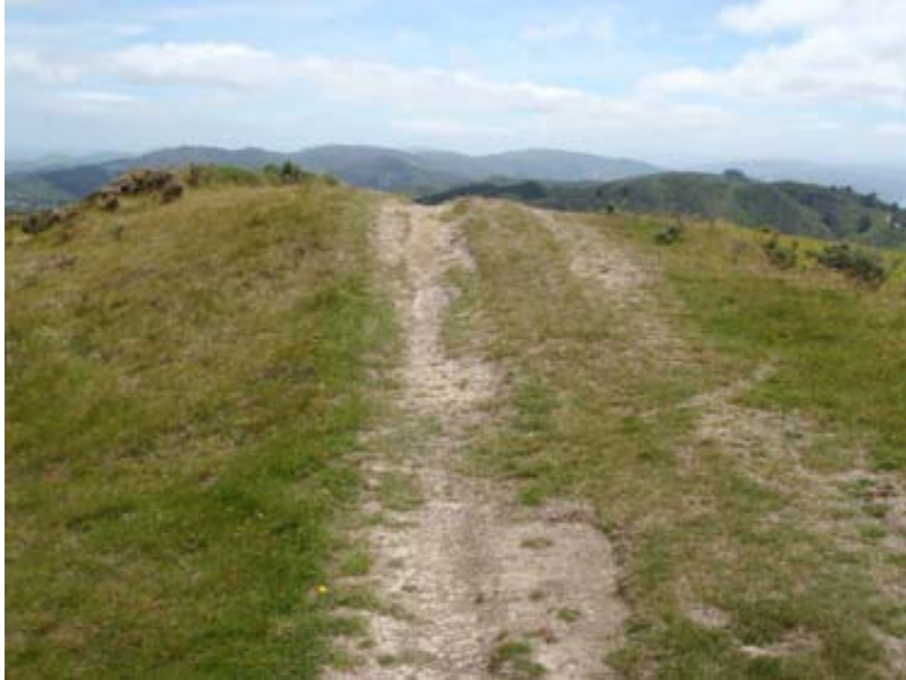
PHOTO 15 – Track access to Turbine 19 – Cut down by 3m
