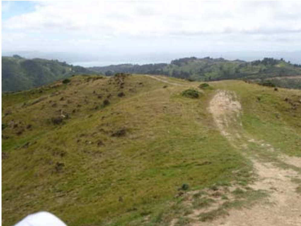
PHOTO 18 – Site of Turbines 19, 20 – Earthworks of vertical alignment required
