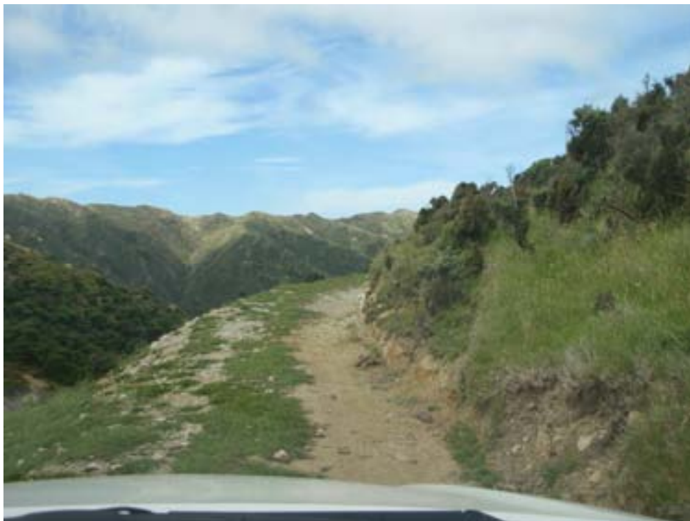
PHOTO 20 – Track to be widened RHS by 3 to 4m
