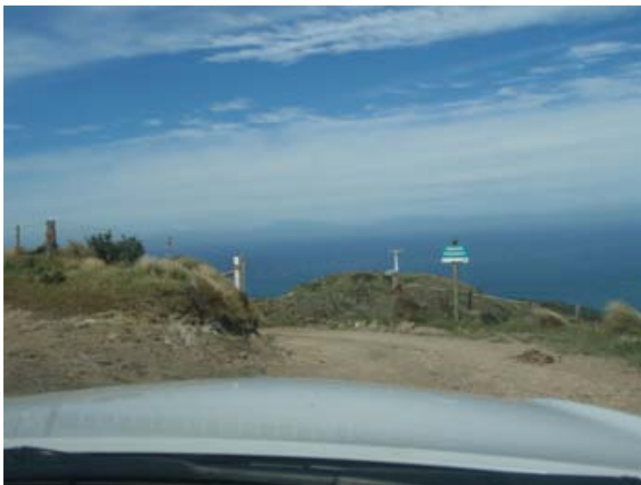
PHOTO 8 – 4 to 5m cut back required on LHS of main track for truck access
