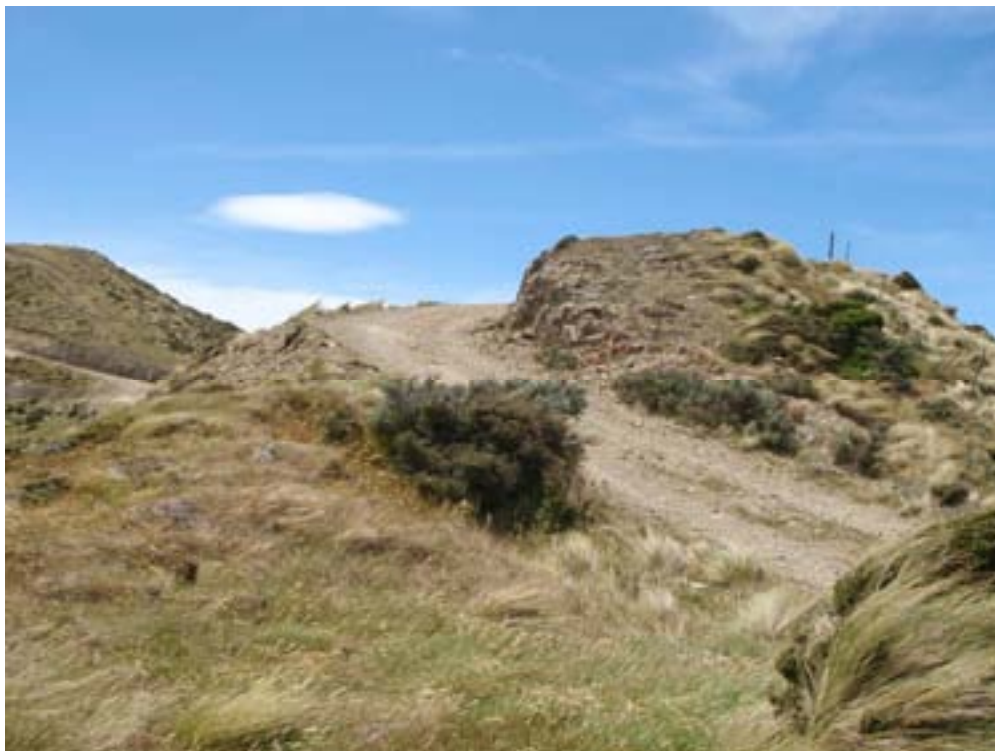
PHOTO 24 – 2m cut back required on RHS of main track for truck access
