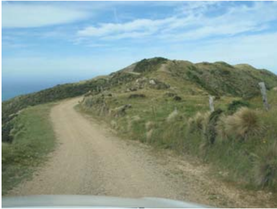
PHOTO 5 – Site of Turbine 5
