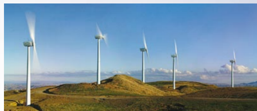
Te Rere Hau wind farm Stage 1
