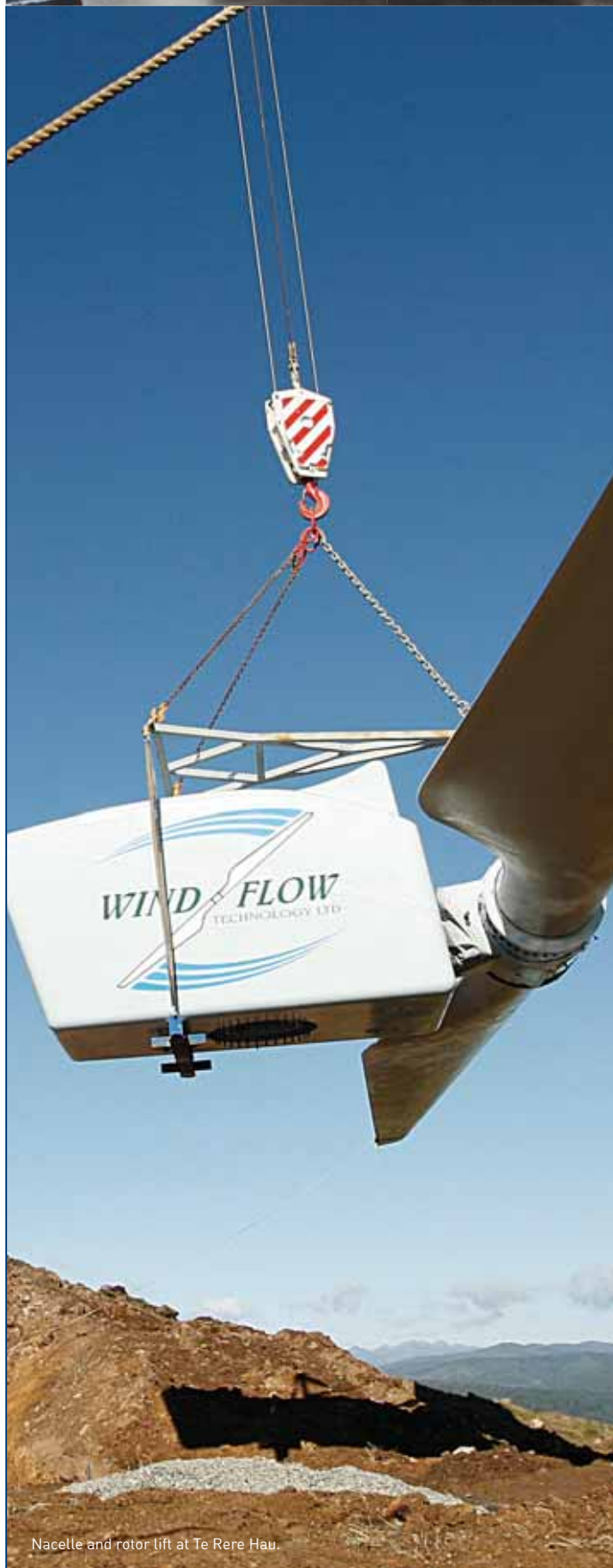
Windflow 500 nacelles being transported to Te Rere Hau.
