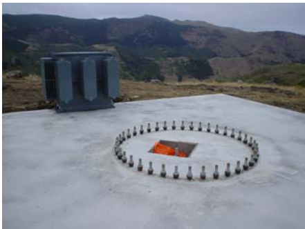
... after pouring, showing the tower base transformer.
